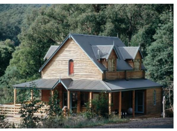
Radially sawn timber weatherboard house
